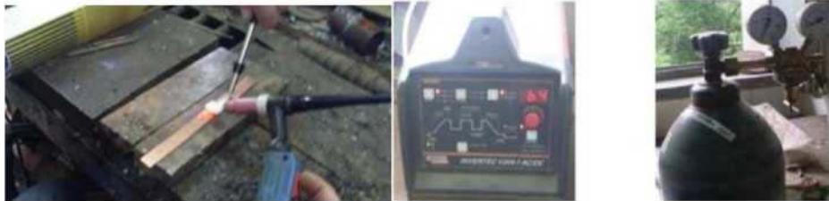
Fig. 37. Installation for TIG welding
